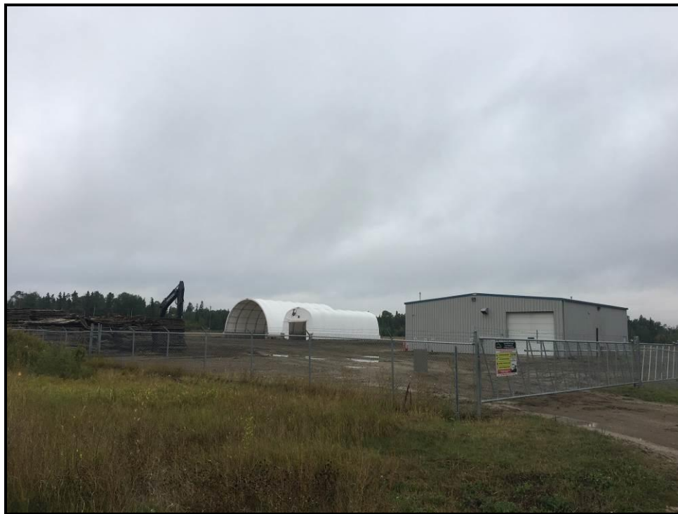
Photograph 1: The Property, as seen from the northeast (September 10, 2018).
