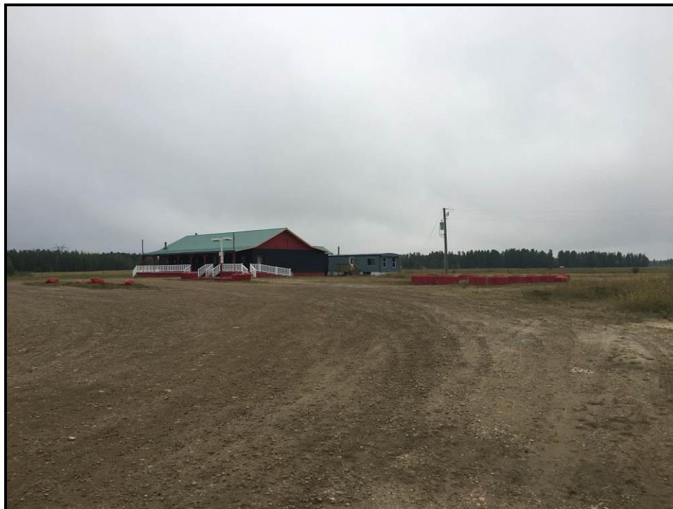
Photograph 8: A former service station to the adjacent east-southeast of the Property (September 10, 2018).
