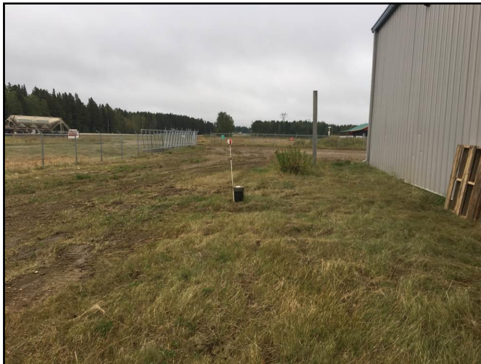
Photograph 4: The septic tank on the northeast side of the shop (September 10, 2018).
