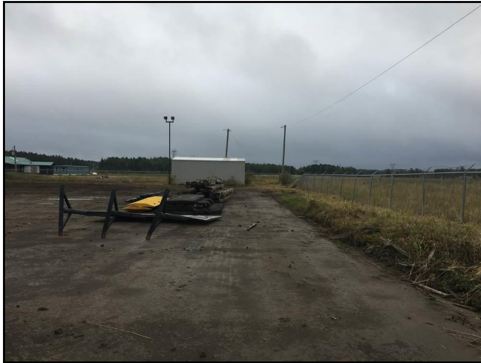
Photograph 7: Miscellaneous storage and an empty shed on the south portion of the Property (September 10, 2018).
