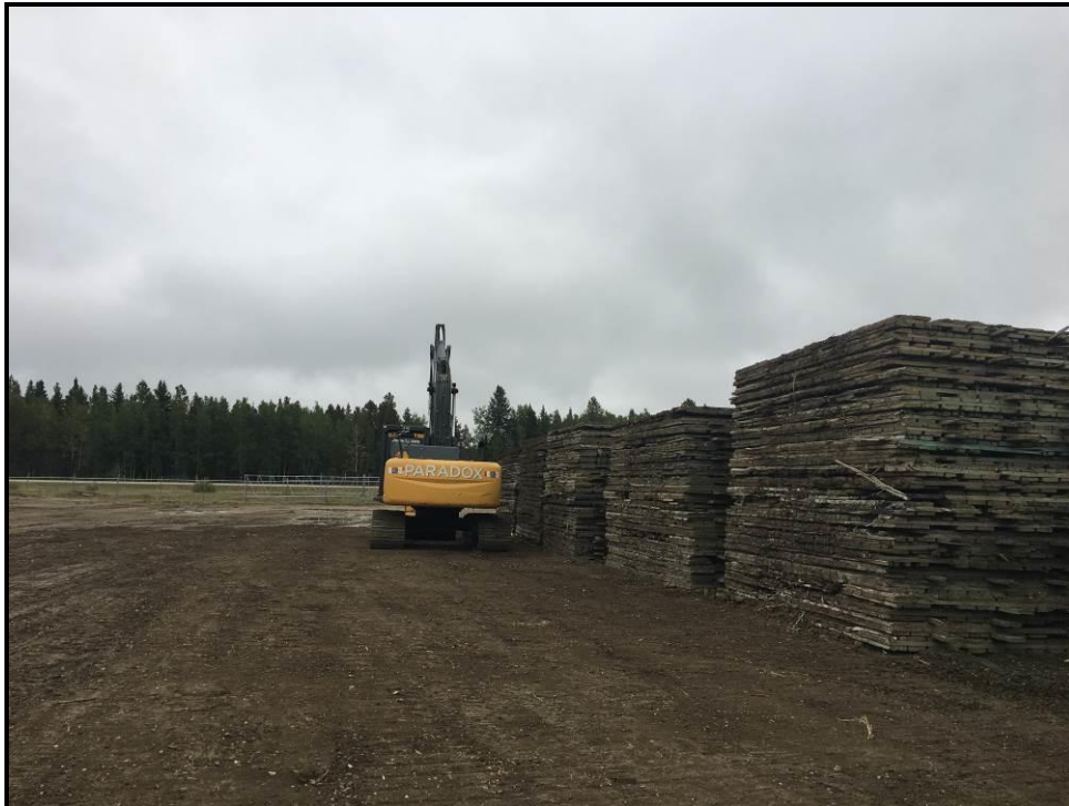
Photograph 6: Rig mat and equipment storage on the east portion of the Property (September 10, 2018).
