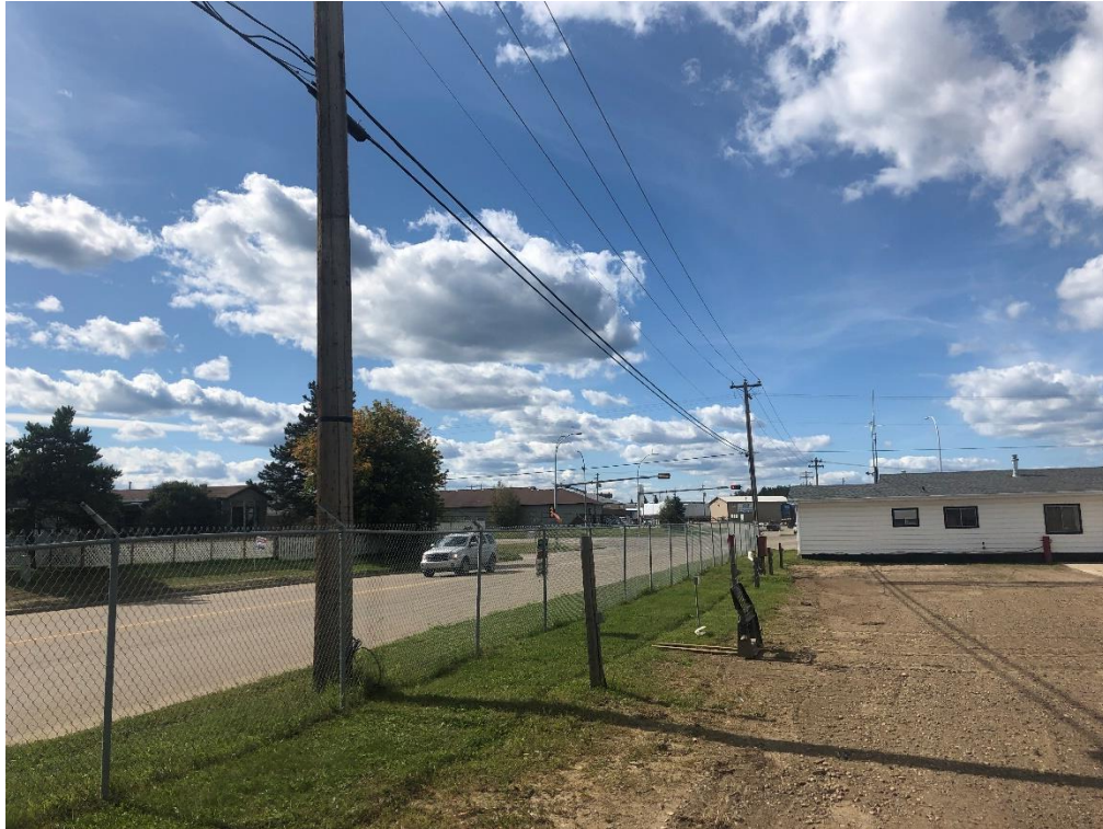
FIGURE 15: SOUTH PROPERTY LINE
