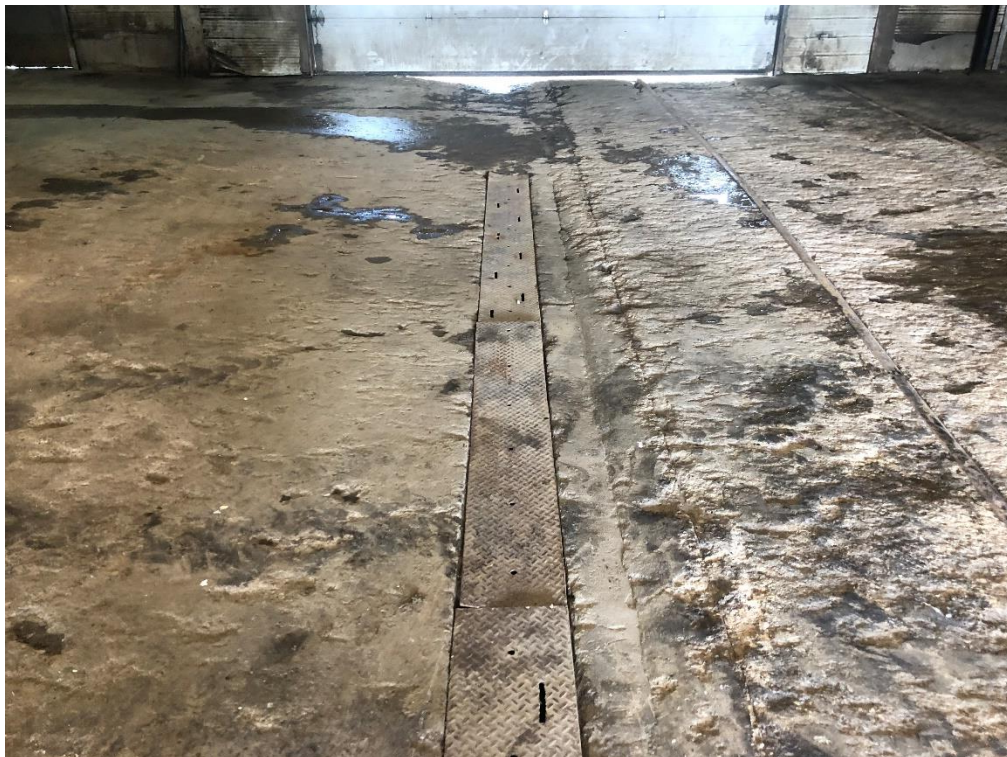
FIGURE 8: TRENCH AND DRAIN IN SECOND SHOP
