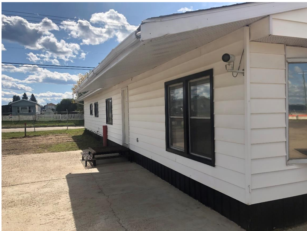
FIGURE 16: OFFICE BUILDING ON SITE
