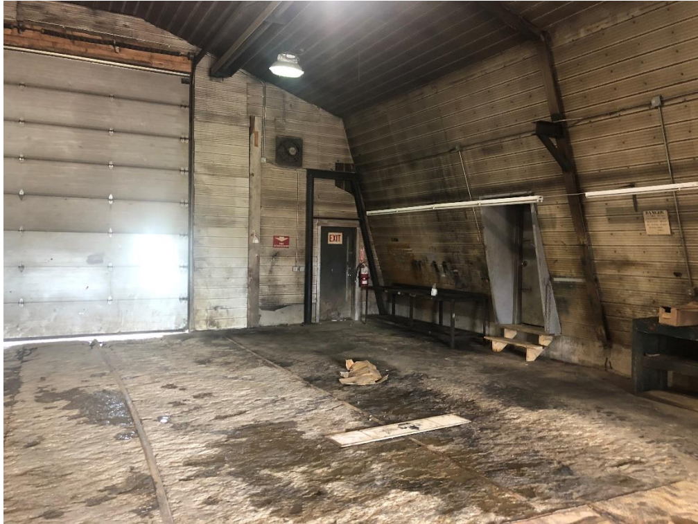
FIGURE 7: SECOND SHOP INTERIOR
