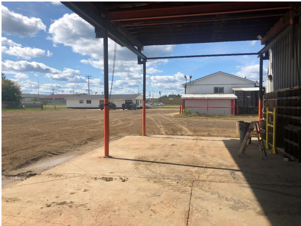
FIGURE 10: CONCRETE PAD ALONG SOUTH SIDE OF SECOND SHOP
