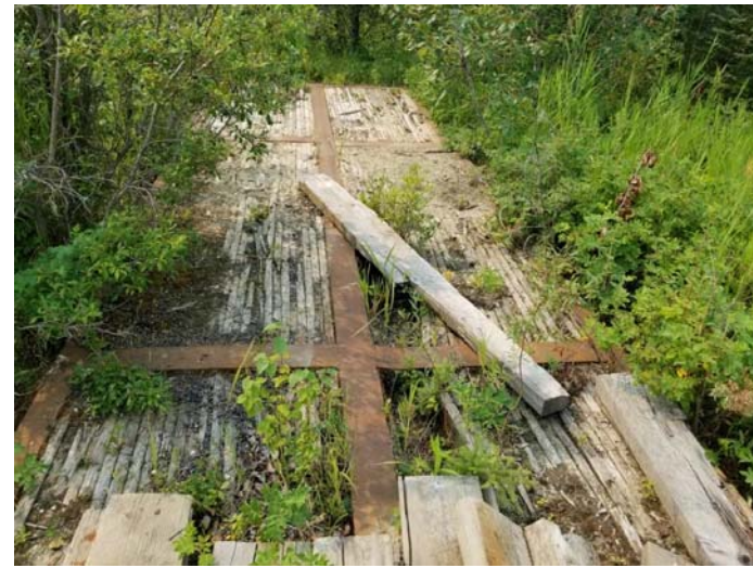
Rig mats on the Site.
