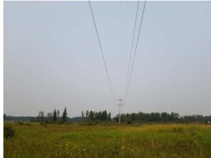
Powerline ROW running from north to south across the Site.
