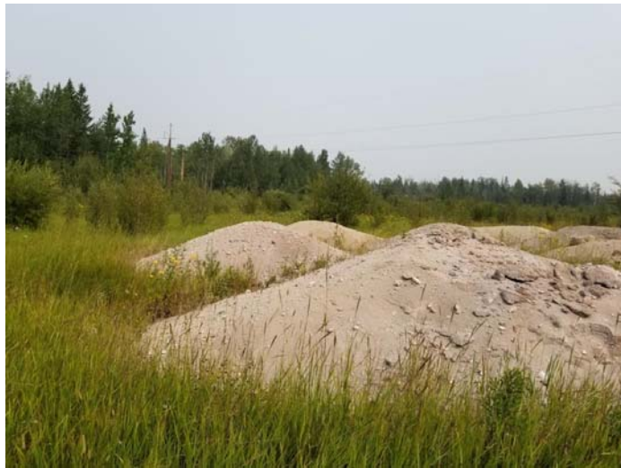
Close-up of sand and gravel piles on the Site.
