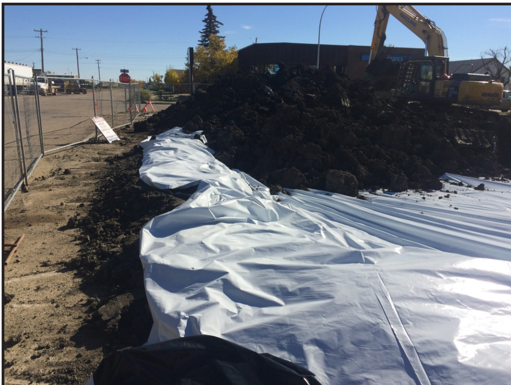
Treatment cell constructed on the north side of the property
