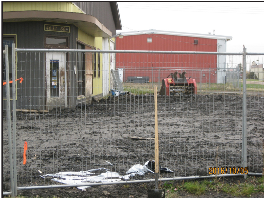
Backfilled north side of property, looking west
