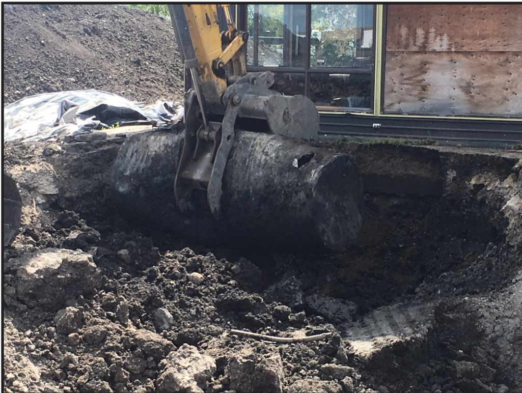
Tank removal from the northeast corner of building
