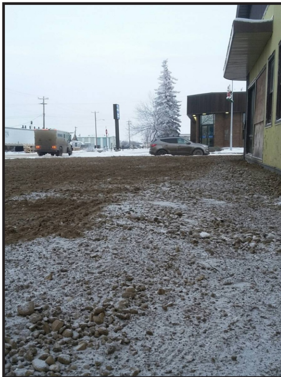
Gravel spread on north side of property facing east
