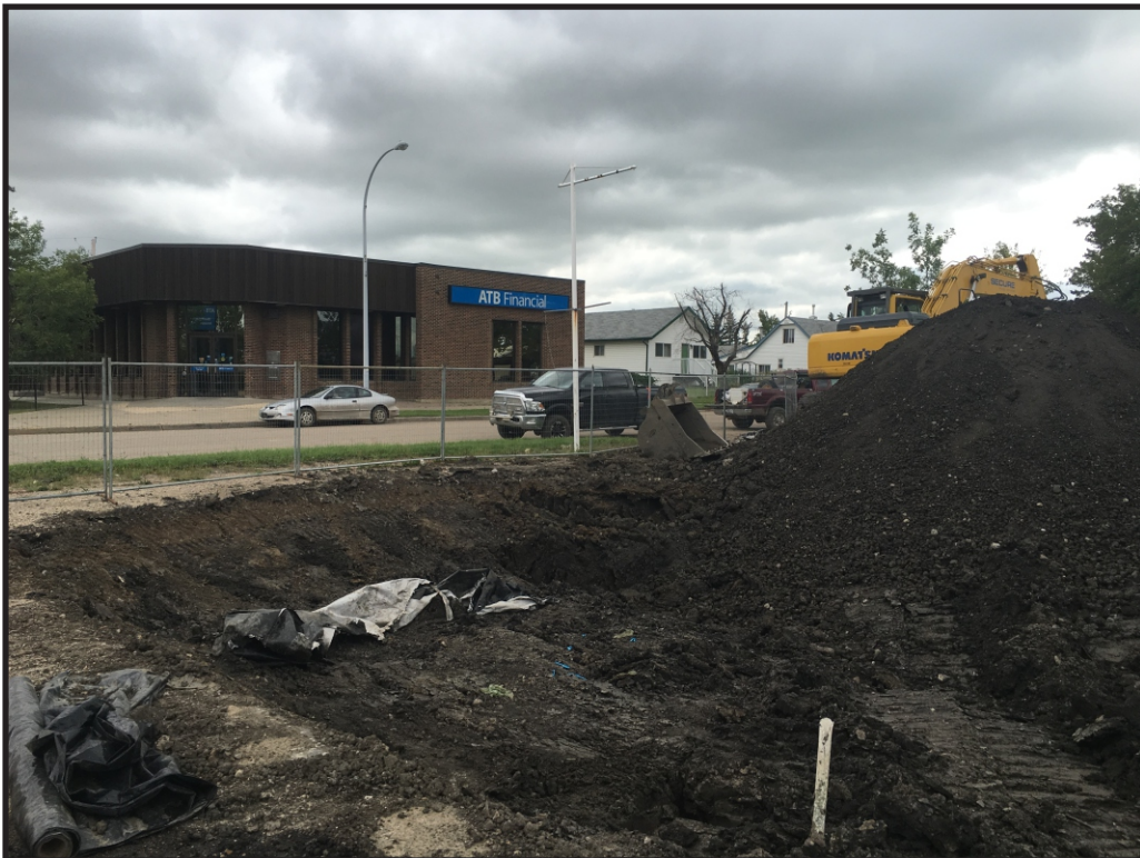
Initial excavation of the north side of property, looking southeast
