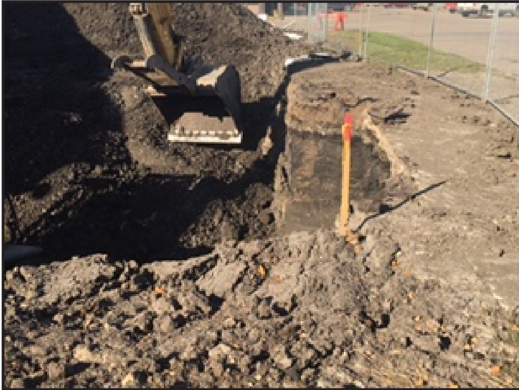
Southeast edge of excavation along south boundary
