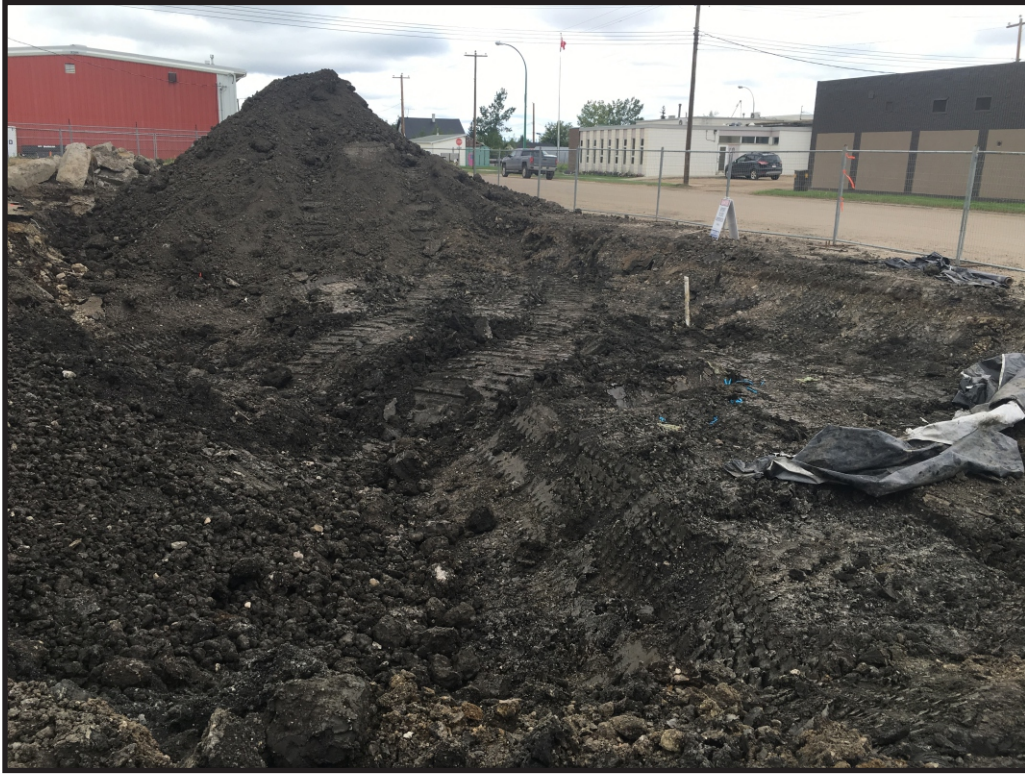
Initial excavation of the north side of property, looking northwest
