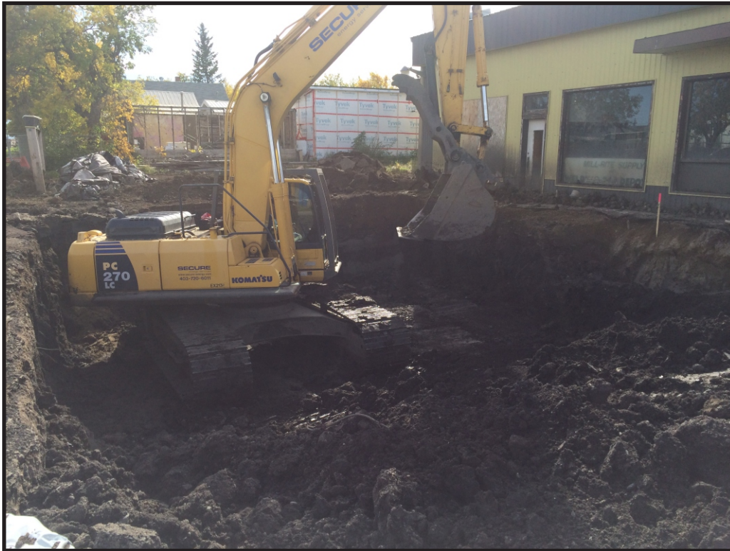
Excavation on west side of property, looking southeast
