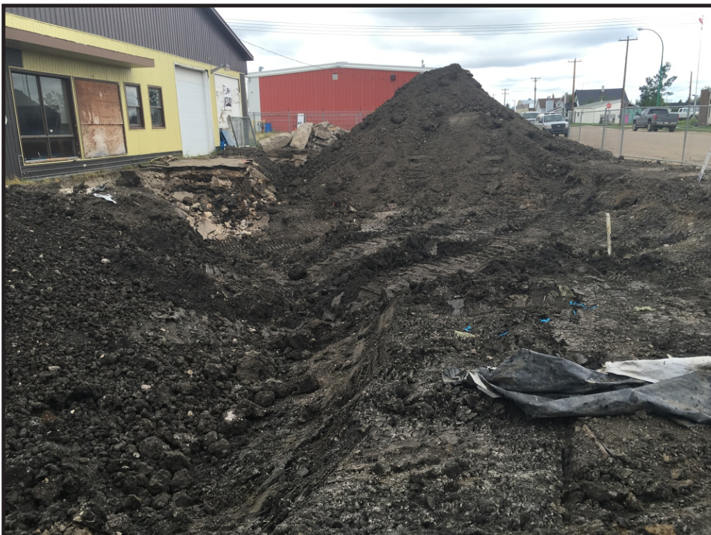
Initial excavation of the north side of property, looking west
