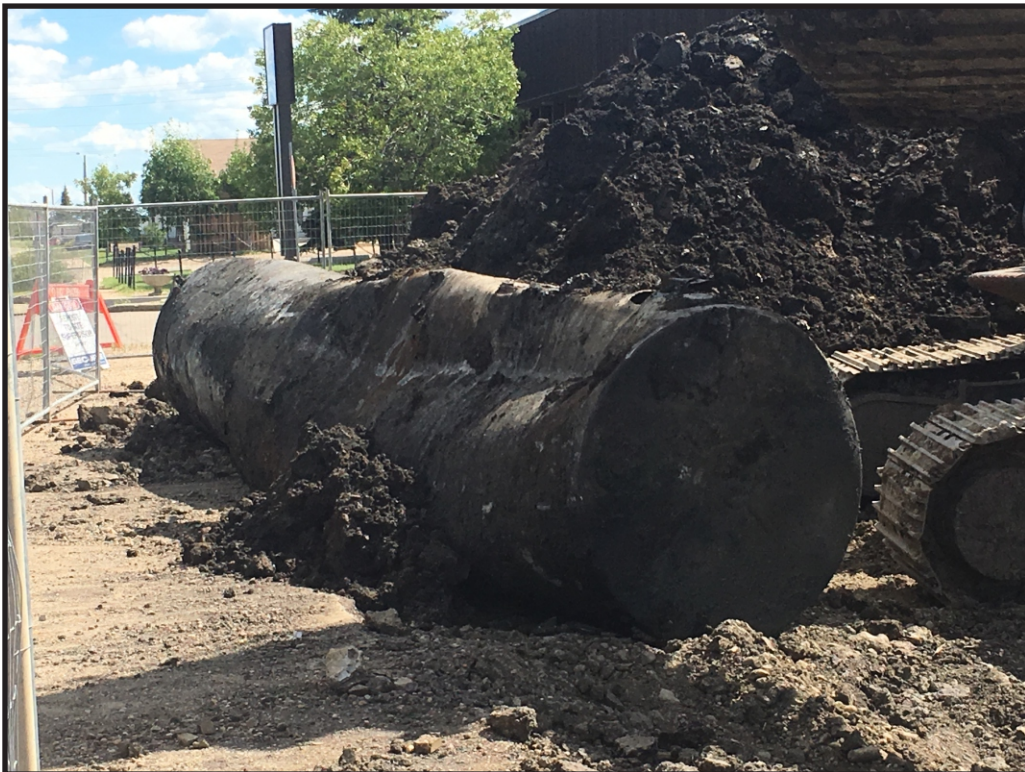
Removed fuel tank
