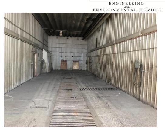
FIGURE 17 – SHOP BAY WITH DRAINAGE SUMP
