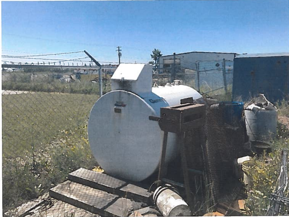
FIGURE 20: EMPTY WASTE OIL TANK
