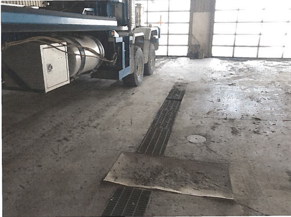
FIGURE 12: SUMP IN SHOP AREA
