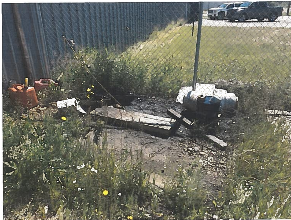
FIGURE 19: SURFICIAL STAINING ALONG WEST BUILDING EXTERIOR
