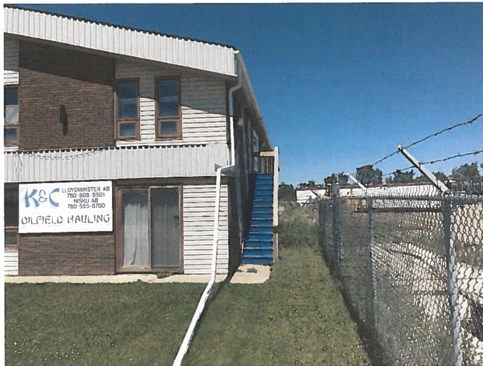
FIGURE 9: EAST BUILDING EXTERIOR
