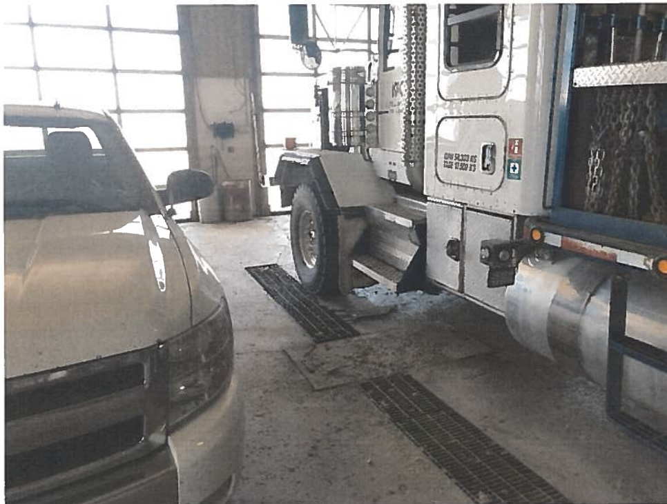
FIGURE 15: SUMP IN SHOP AREA
