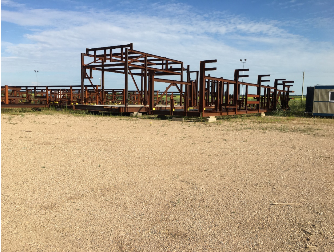
Photo 3: View of module frames stored on the Site.
