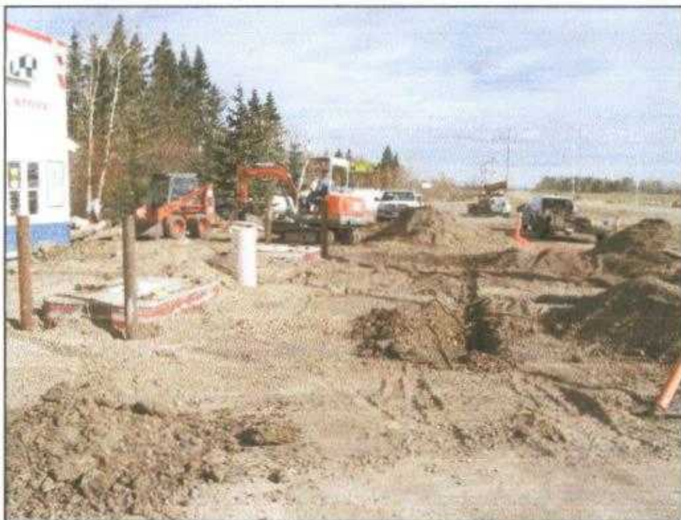
Photograph 8: Site # 5720 – View looking east after backfilling.
