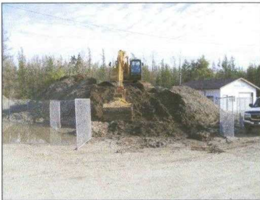
Photograph 6: Site # 5720 – Contaminated soil being aerated with allu bucket at east end of site.
