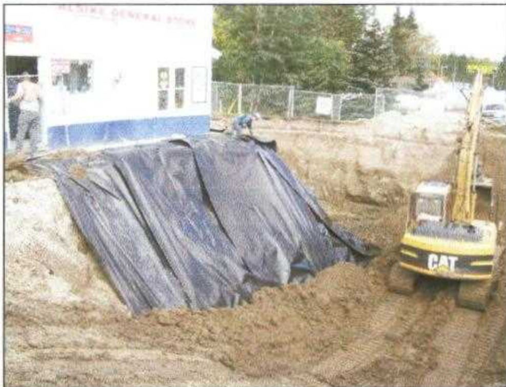
Photograph 7: Site # 5720 – Installation of Geo-membrane liner.
