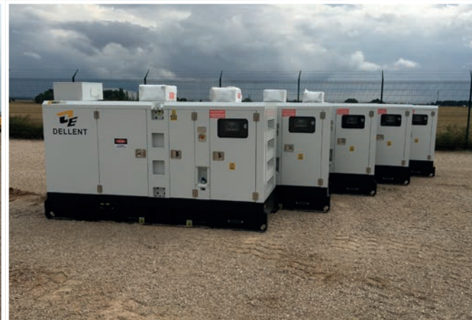
5 - UNUSED — 2020 DELANT GF2-120 150 KVA
