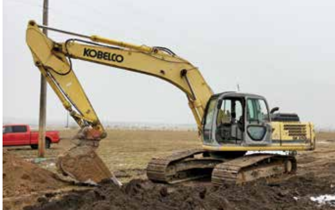
1 of 4 – Kobelco SK250LC
