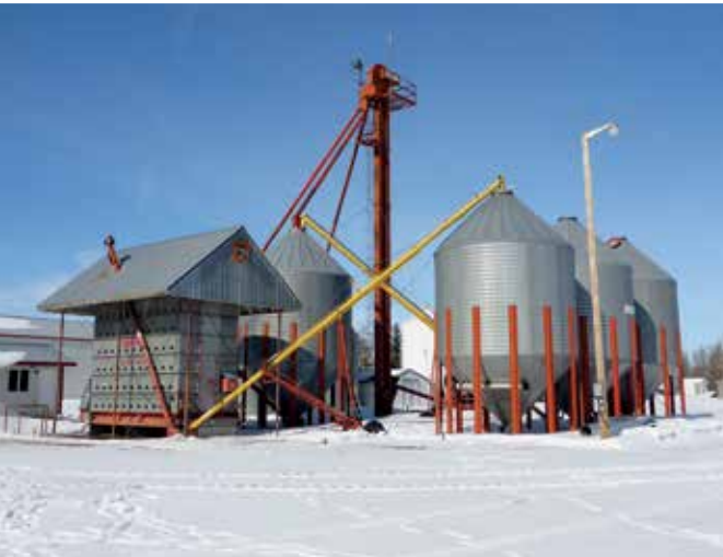
Vertec VT6600 Dryer, Behlen Bins, Behlen 60 Ft Leg & Westfield Augers
